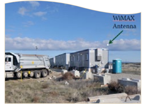
WiMAX is saving the environment and allowing for faster deployment of telecommunications abilities throughout the Hanford Site.
