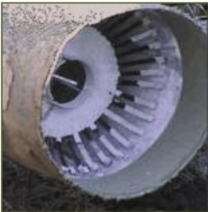
*Mortar lining, a new technology, is being used to refurbish ~28 miles of water lines.*
