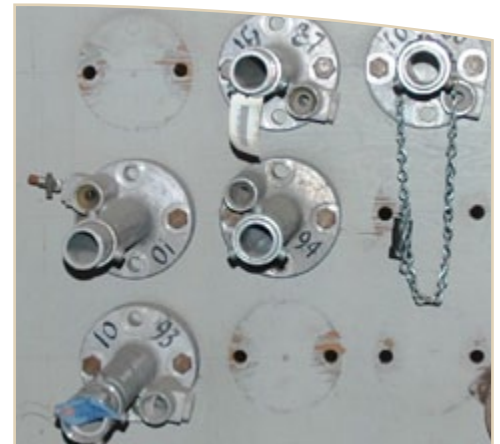
Manhattan Project-era nuclear reactor nozzles
